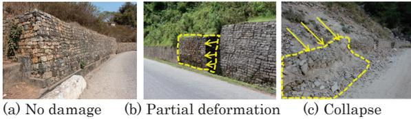
Fig. 1 Classification of damage types of retaining wall along Asian highway 42<sup>6)</sup>.
